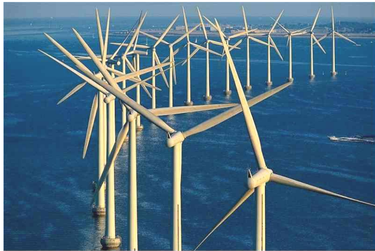
Offshore electric windmill generators.
